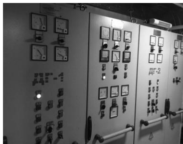
Figure 2 – The switchboard is divided into several sections: section 1 - diesel generator 1; section 2 - synchronization and power from the shore; section 3 – diesel generator 2; section 4 - load bus 3F, 230V, 50 Hz.
