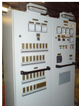
Figure 1 – The emergency switchboard
